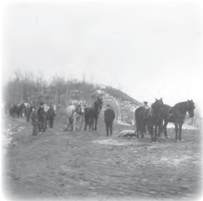
Saskatchewan Hospital Road Construction 1915 (credit: The City of North Battleford Historic Archives)
