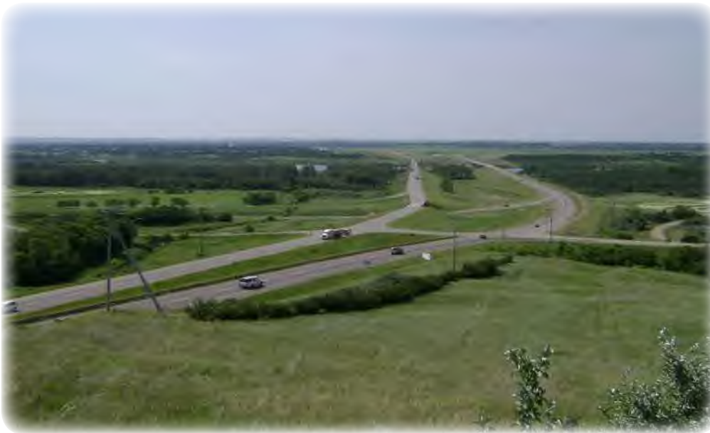
Highway 4/16 at King Hill Lookout (credit: AECOM)
