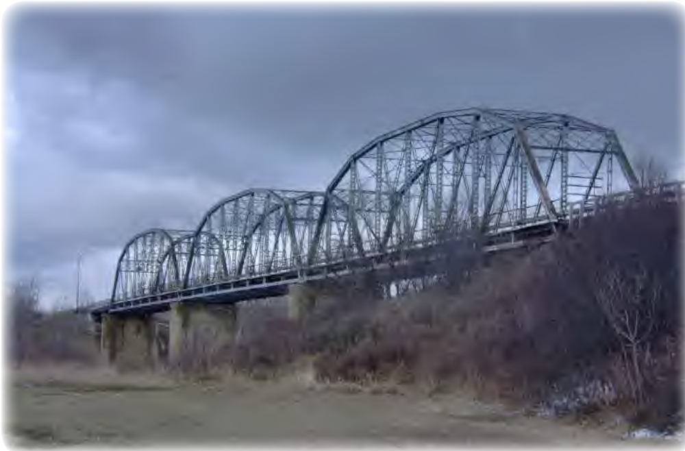
South Open Traffic Bridge on Finlayson Island
