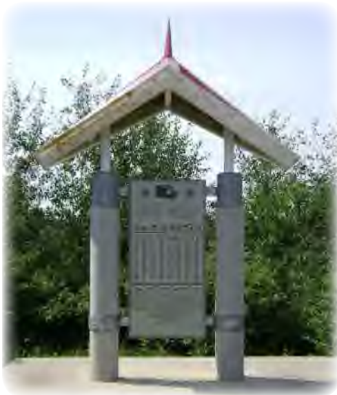
Trans Canada Trail Pavilion (credit: AECOM)
