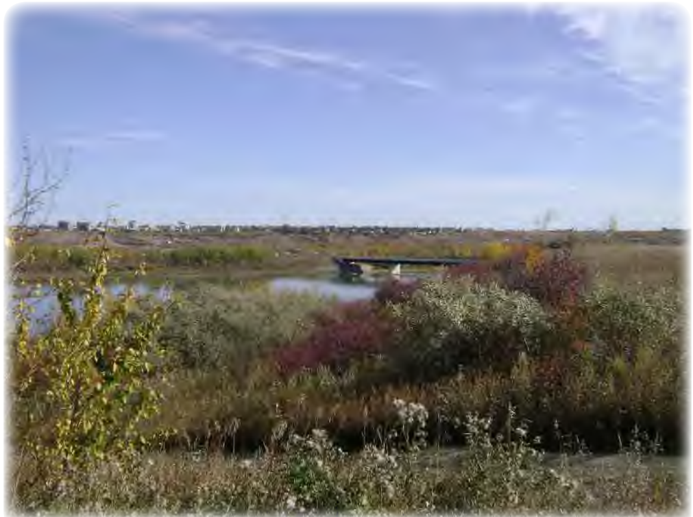
Looking downstream towards North Battleford (credit: AECOM)
