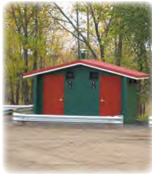
Brick washrooms and parking improvements, Finlayson Island, built in 2008
